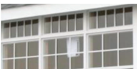
Transom Windows (above windows)
